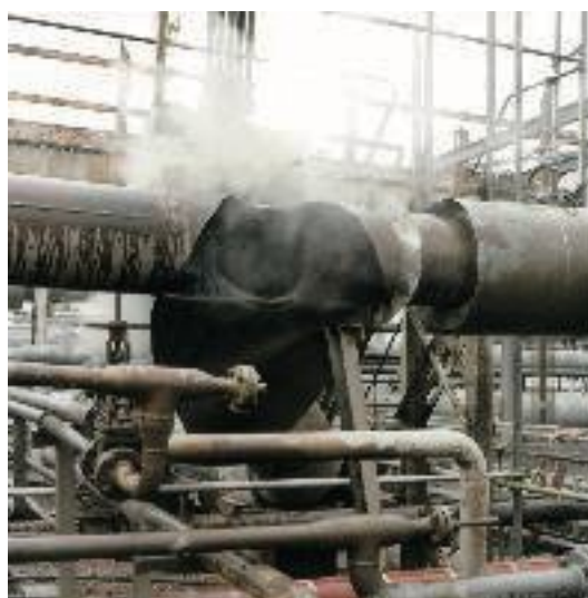
▲ Fig. 12. Significant blow-out of a steam pipe due to a water hammer event (BP Grangemouth, 2000).
